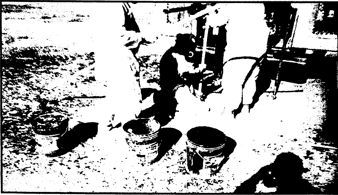
Installation of piezometer GP-99-18.
