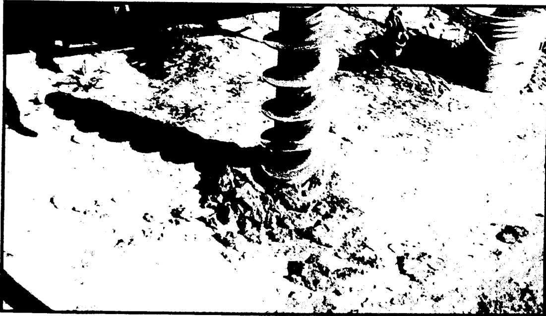
MSW augered to the surface during installation of deep boring DB-1.
