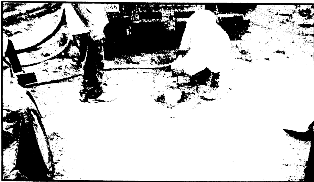
Plugging of DB-3 by placement of grout to the surface.
