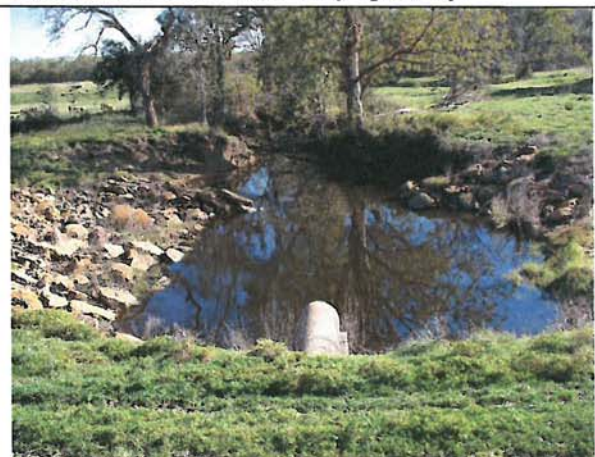
Outlet pipe, stilling basin, and outlet channel. Scour erosion on both sides of channel just past the rock riprap.
