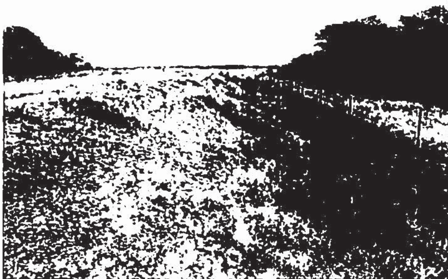
Photo 12: Downstream slope from the right end, view to the east. Note the large bare areas along the downstream slope.
