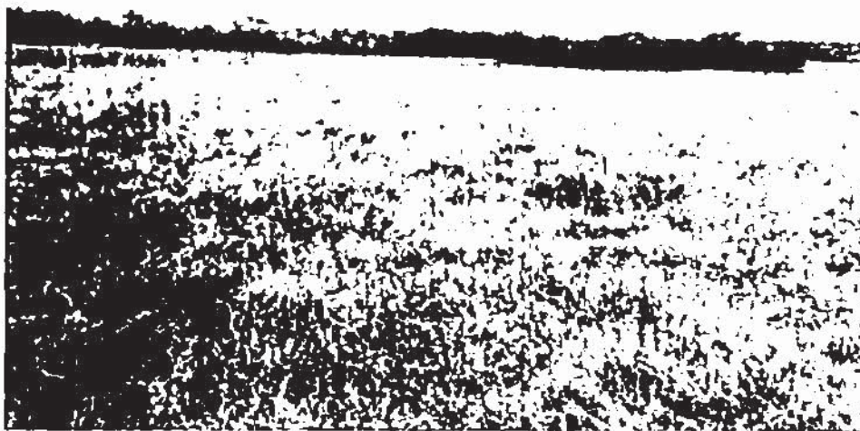
Photo 24: Emergency spillway exit channel, looking southwest. Note the well-established and tall grass cover that is generally clear of trees and vegetation. Trees are noted at the end of the channel.
