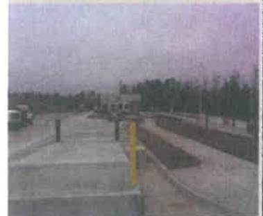
Construction underway on scale house
