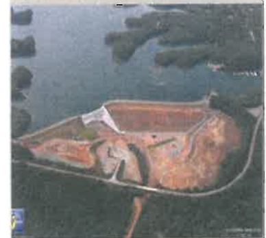
Completed Catawba Dam Stabilization Project for Duke Power
