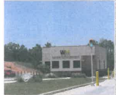
Energy-efficient administration building at Turkey Run
