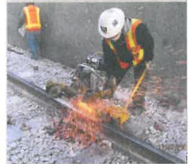
Herzog worker destresses rails after welding
