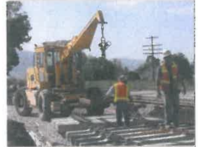
Cross tie installation by Herzog
