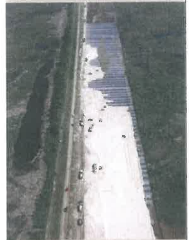
Levee Modifications in New Orleans
