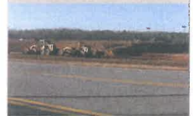
Construction underway at Mando Corp.
