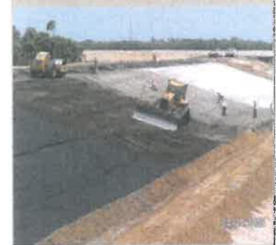
Construction of Ten Mile Creek Reservoir
