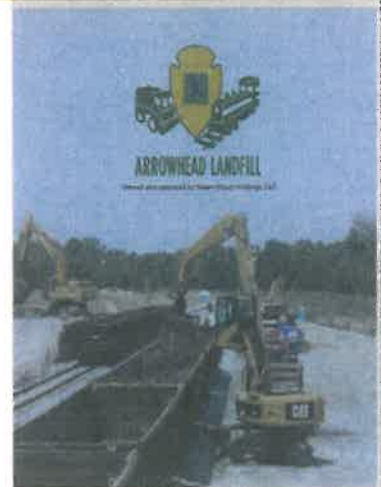
Arrowhead Landfill Uniontown, Alabama
