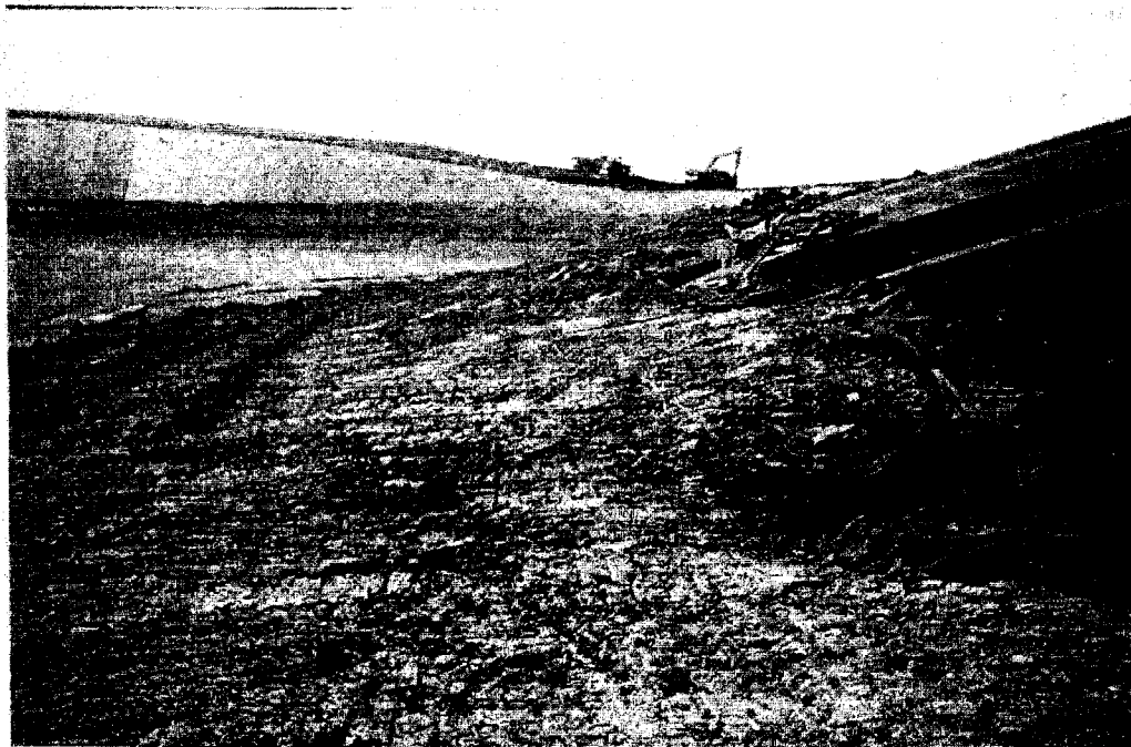
Cell WD-3 Northwest Sideslope Geonet/Geotextile Slippage Area at Toe of Slope Prior to Repair View Toward South January 5, 1999
