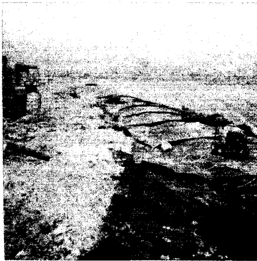
Cell WD-3 Northwest Sideslope Geonet/Geotextile Slippage Area at Top of Slope Prior to Repair View Toward North January 5, 1999
