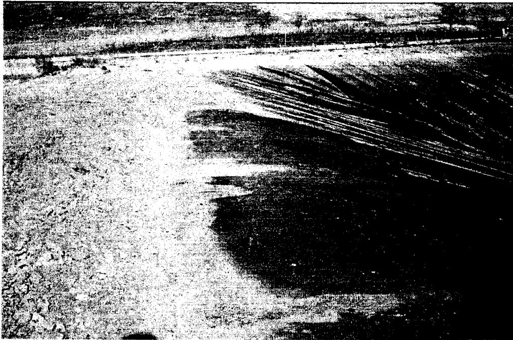
Cell WD-3 Northwest Sideslope Geonet/Geotextile Slippage Area at Top of Slope Prior to Repair View Toward North January 5, 1999
