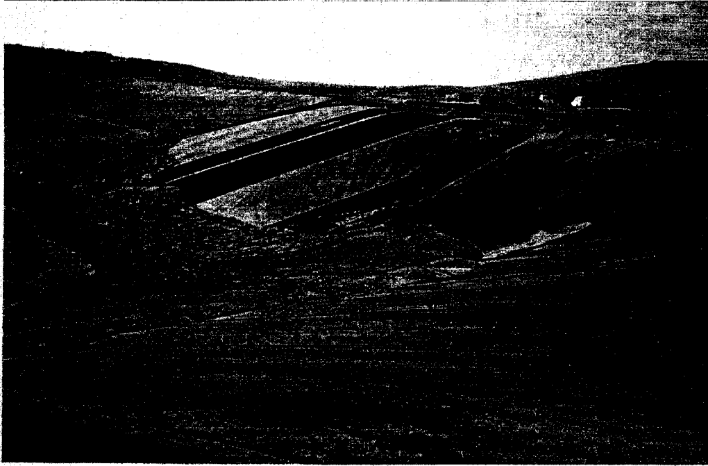
Cell WD-3 Northwest Sideslope Geonet/Geotextile Slippage Area Prior to Repair View Toward Southwest January 5, 1999
