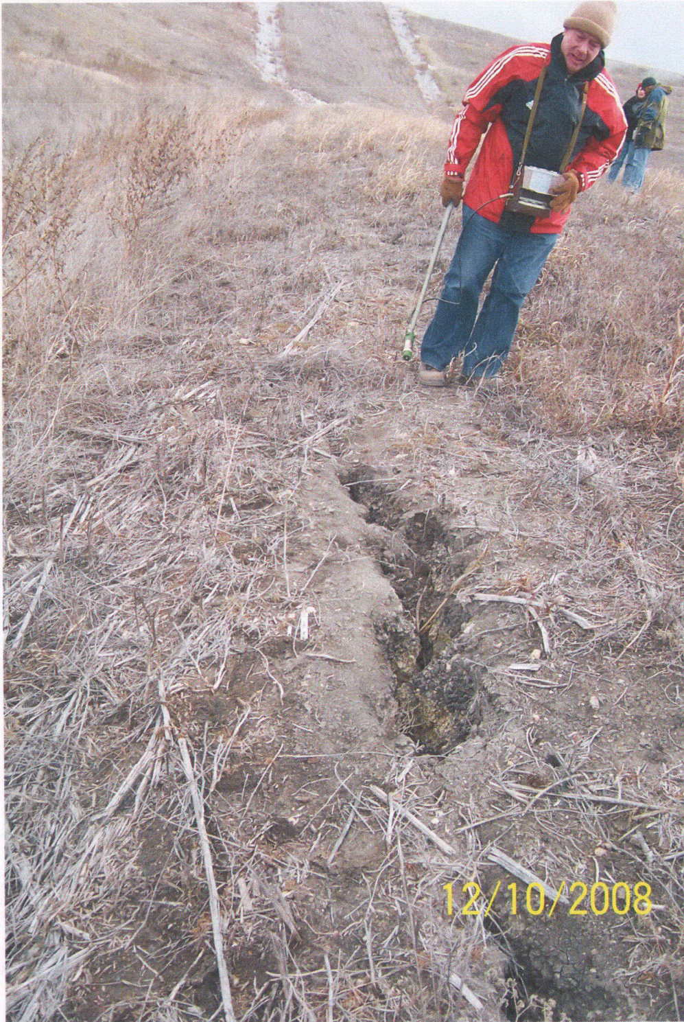
A “tension crack” on the north side of the IWU at the top of the slope.
