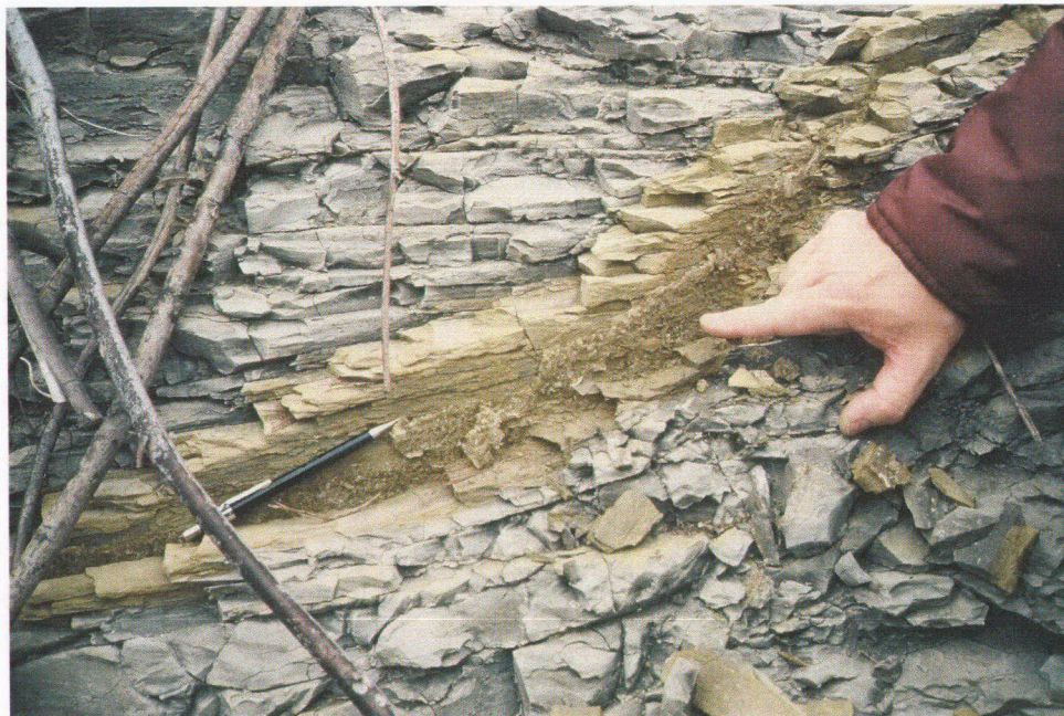
Exhibit TJFA 424-B, Mineralization in Joint in Weathered Taylor Marl – Skyline MSW Landfill
