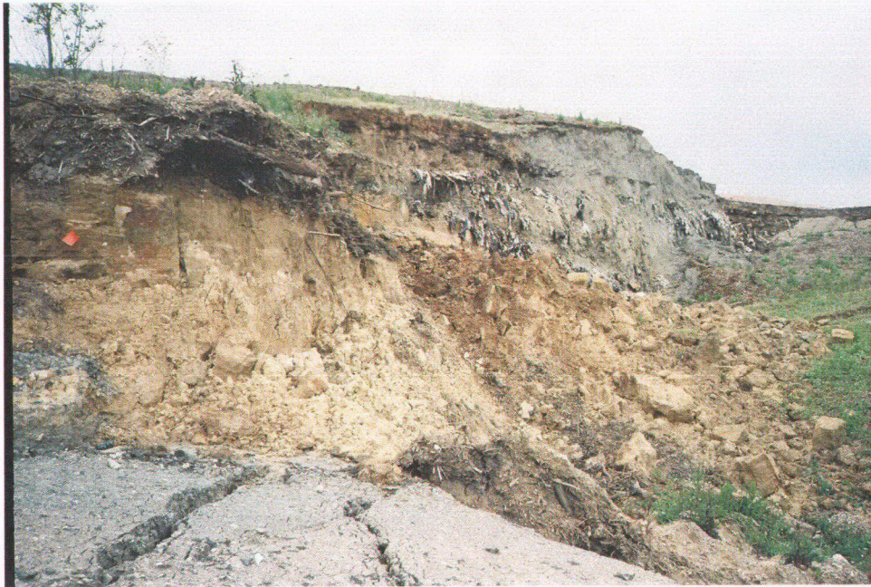
Exhibit TJFA 424-J, Excavation Slope Failure – City of Irving MSW Landfill, 1999
