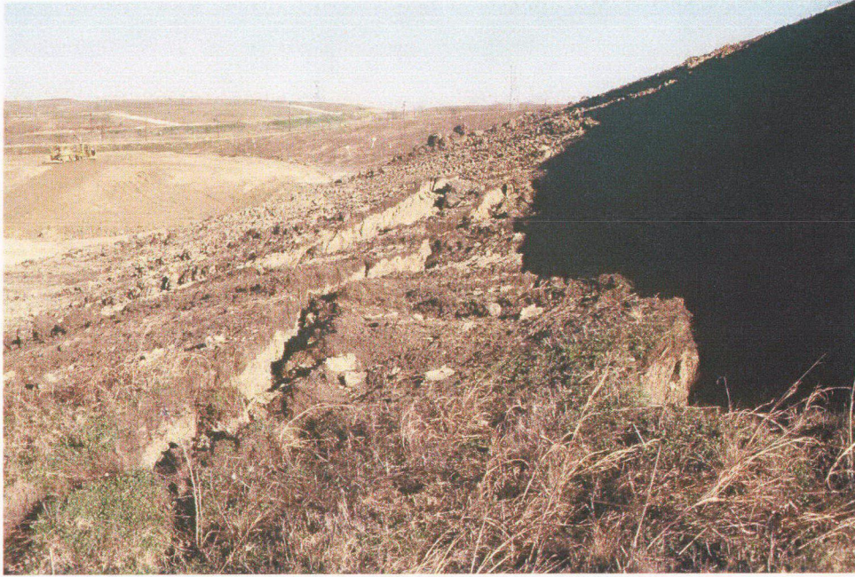
Exhibit TJFA 424-F, Excavation Slope Failure – Skyline MSW Landfill, 1999
