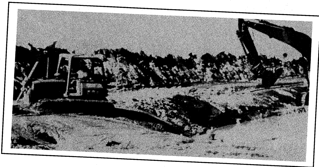
Figure 7.12 - Mixing Backfill with Bentonite Slurry.
