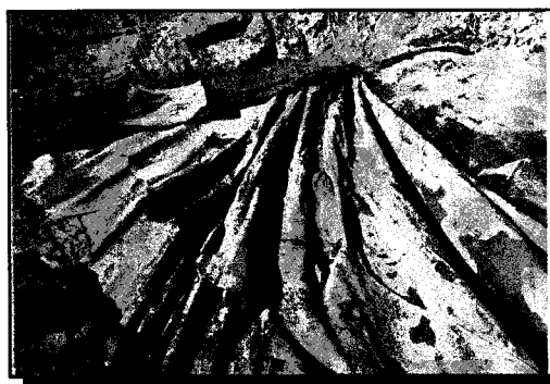
Figure 8-8 Damage to FML of an Ohio landfill at the bottom of a slope from a deep-seated translational failure involving RSL and unreinforced GCL. Contrast this with the tension crack near the top of the same slope shown Figure 8-7 .
